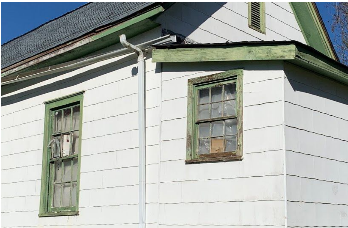
Fig. 9c: Small Six-over-six Wood Sash Window (1903)
