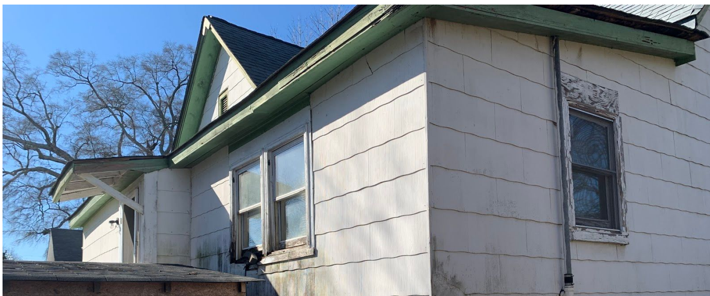
Fig. 9c: Small Six-over-six Wood Sash Window (1903)
