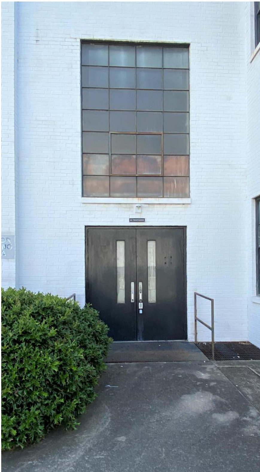
Fig. 11a: Four-over-seven Metal Framed Casement Windows
