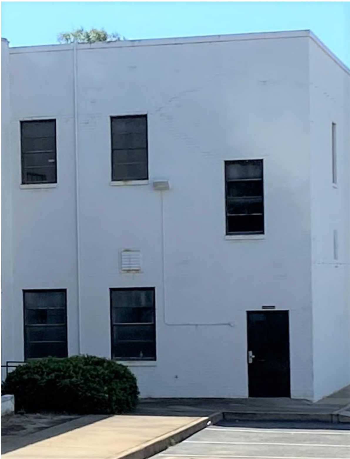
Fig. 11c: Two-over-two metal framed windows
