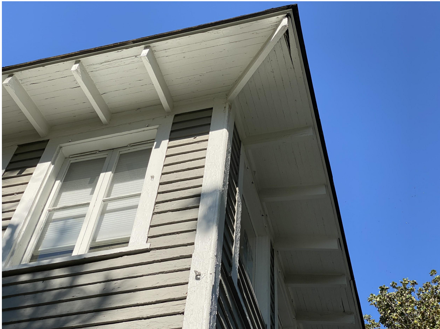
Fig. 8: Deep, bracketed eaves
