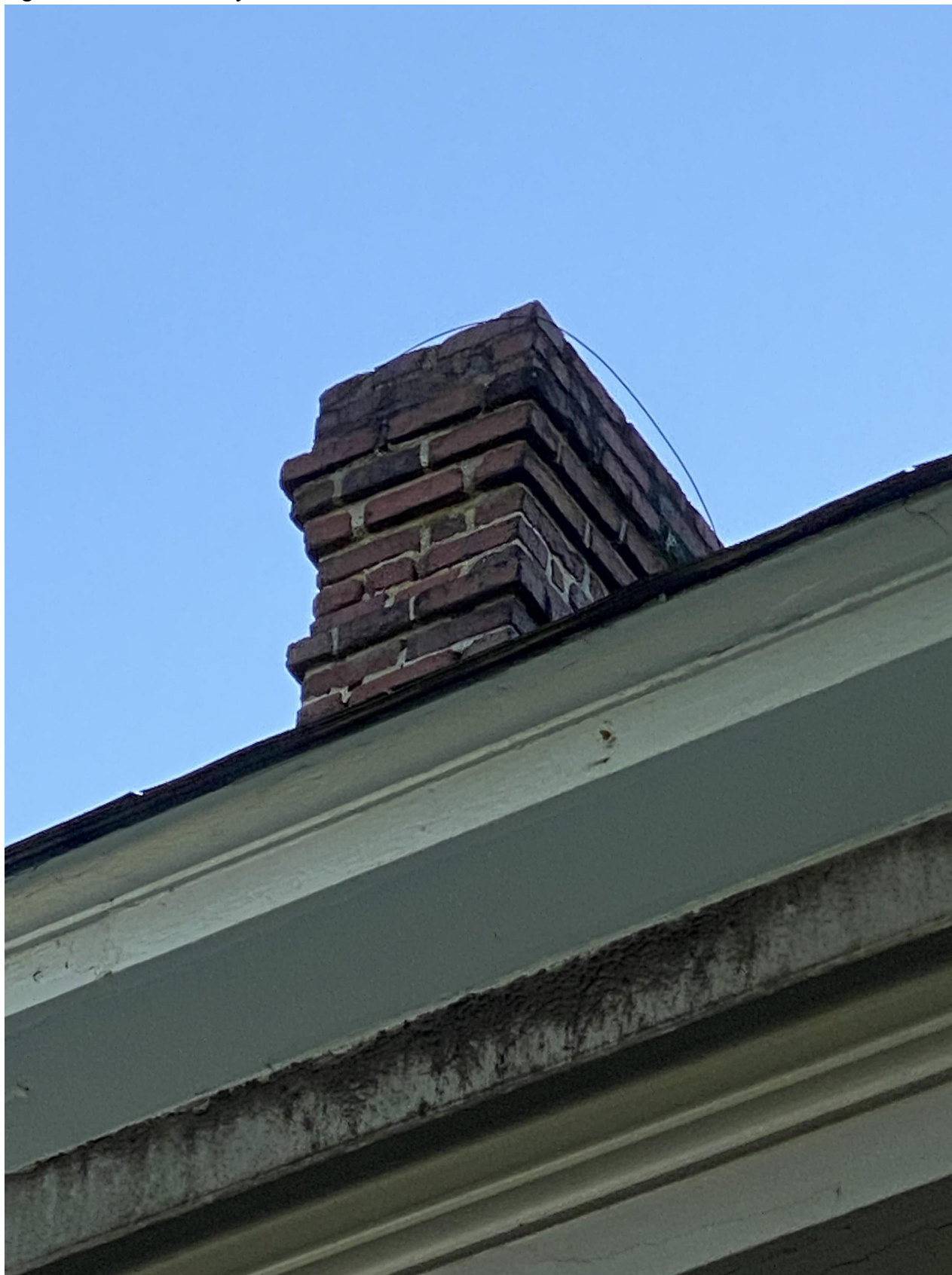
Fig. 9: Corbeled chimney
