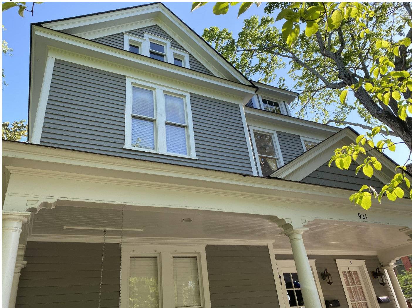
Fig. 7: Pedimented eaves
