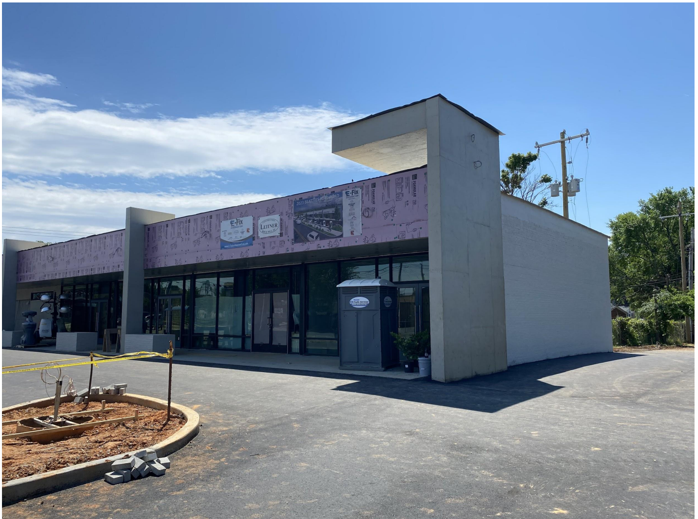
Figure 5: Side (west) elevation facing Taylor Avenue
