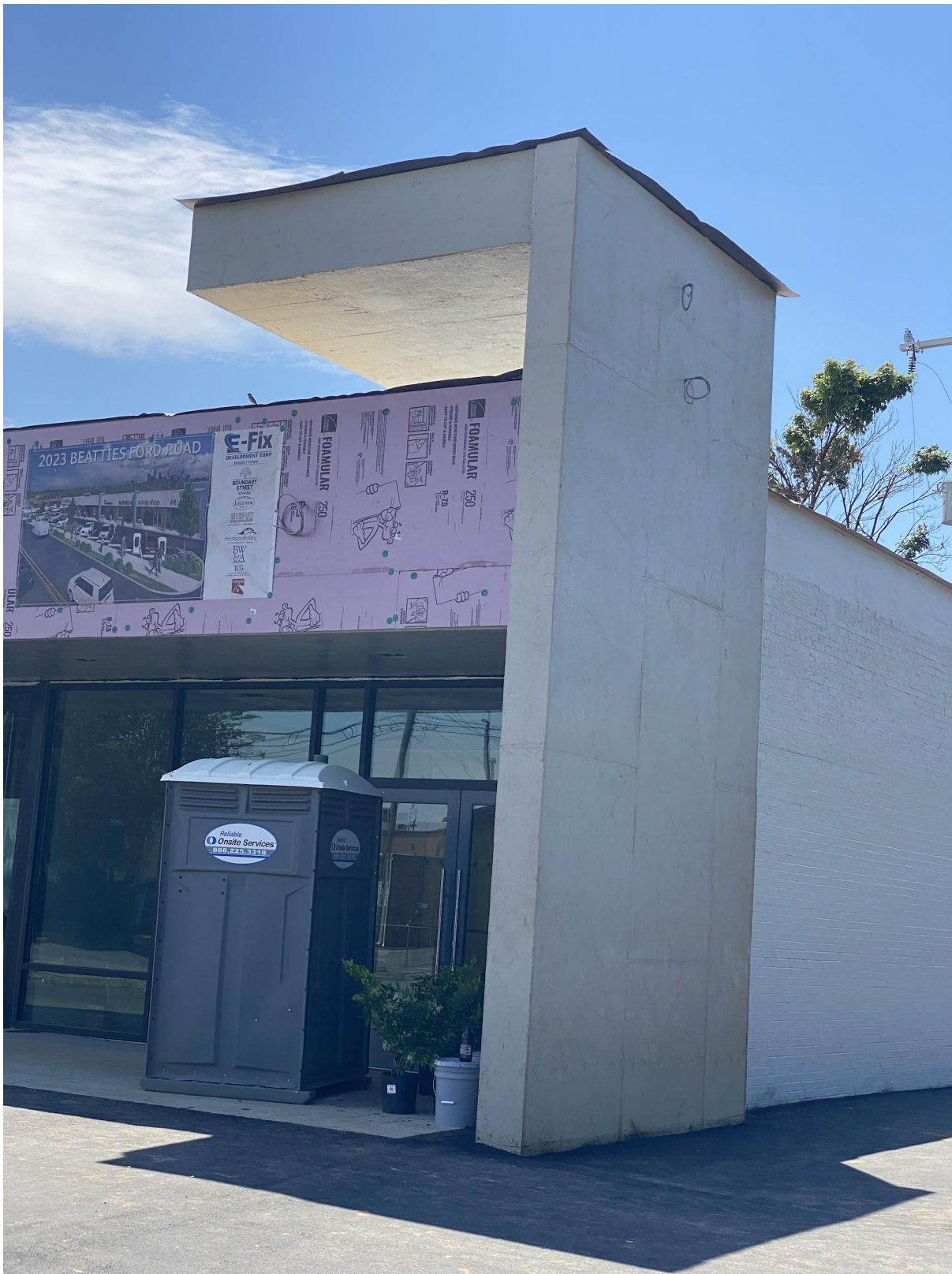
Figure 10: Concrete canopy to west
