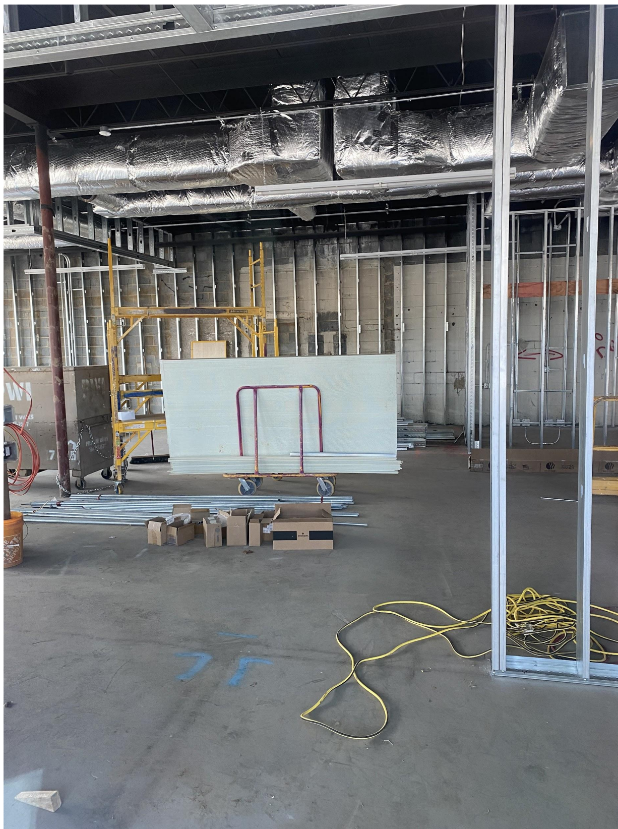
Figure 13: Interior under construction
